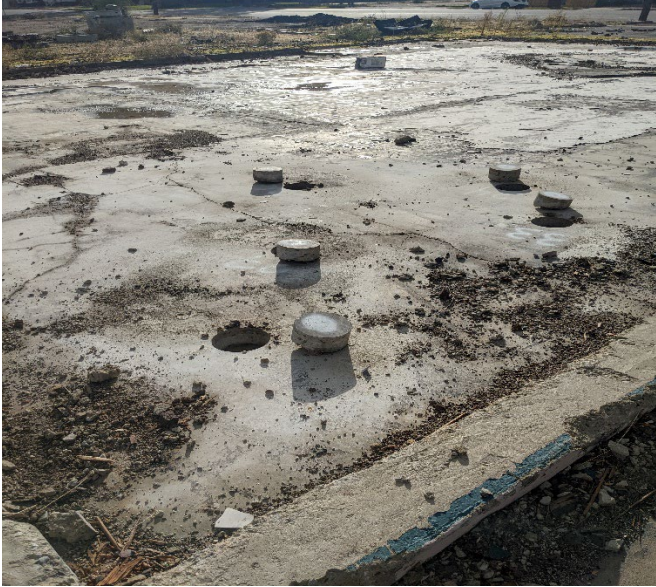
Photo # 1: Openings in the slabs for new well borings.
