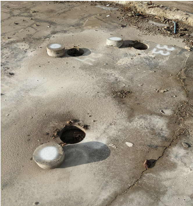
Photo # 2: Boring openings.
